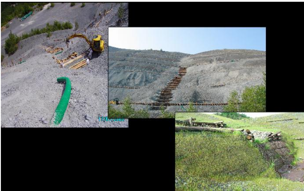
Fig. 2 Various phases of the environmental rehabilitation work.
